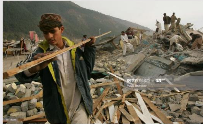
a worker helps to clear the debris.
