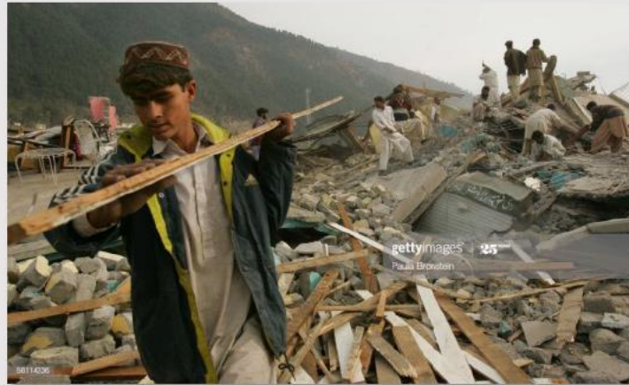
a worker helps to clear the debris.
