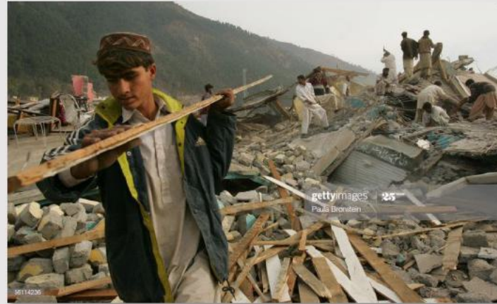
a worker helps to clear the debris.
